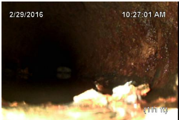
2/29/2016 10:27:02 AM Connection-Cleanout E. 12 o'clock. End continuous surface roughness. End inspection.
