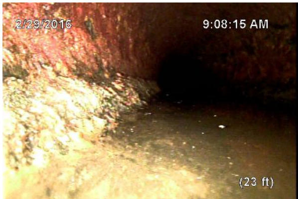
2/29/2016 9:08:16 AM SRI - surface roughness increasing
