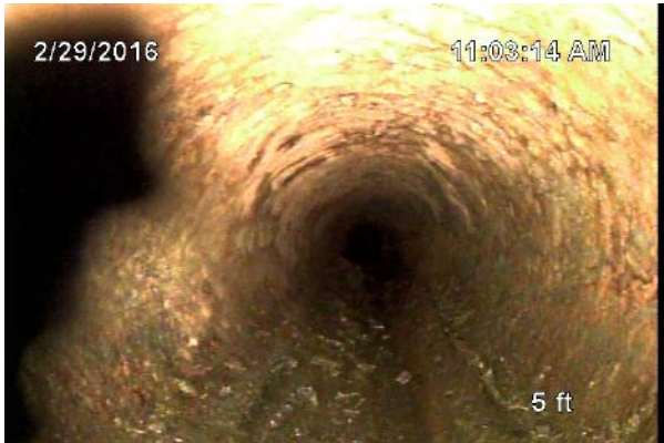
2/29/2016 11:03:15 AM CL - Linear crack
