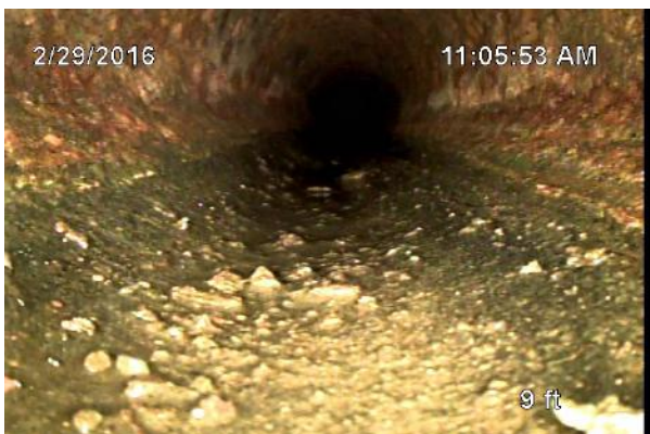
2/29/2016 11:05:53 AM CL - Linear crack
