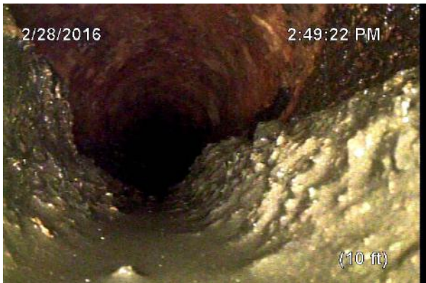
2/28/2016 2:49:23 PM 90 degree bend-turns horizontal.
