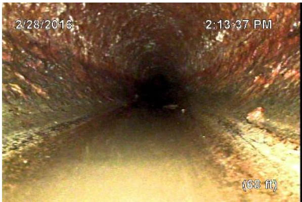
2/28/2016 2:13:38 PM CL - Linear crack
