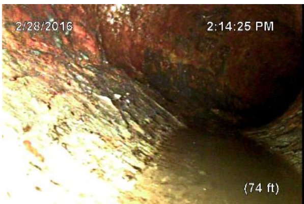
2/28/2016 2:14:26 PM SCP - surface corrosion present - end continuous.
